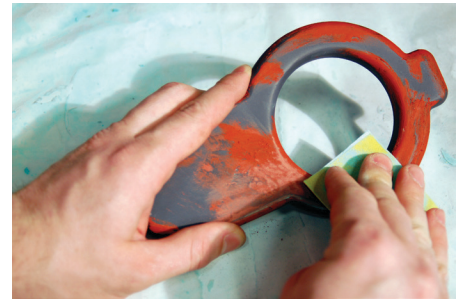
Figure 27 Sand the filler after it has dried.
